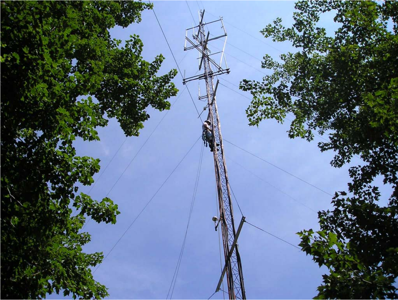
Our intrepid climber, Chuck - N1KGY, in position on the tower.
